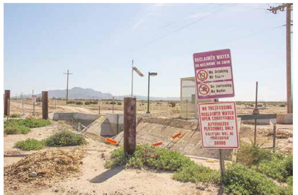
Christopher Lomahquahu/GRIN Purple signs indicate the presence of reclaimed water, which is used for agriculture, dust control and other applications.
