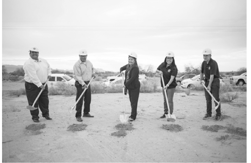
Community Council Representatives and members from GRICUA break ground on the Sacaton Substation 2 on Aug. 15. Christopher Lomahquahu/GRIN
