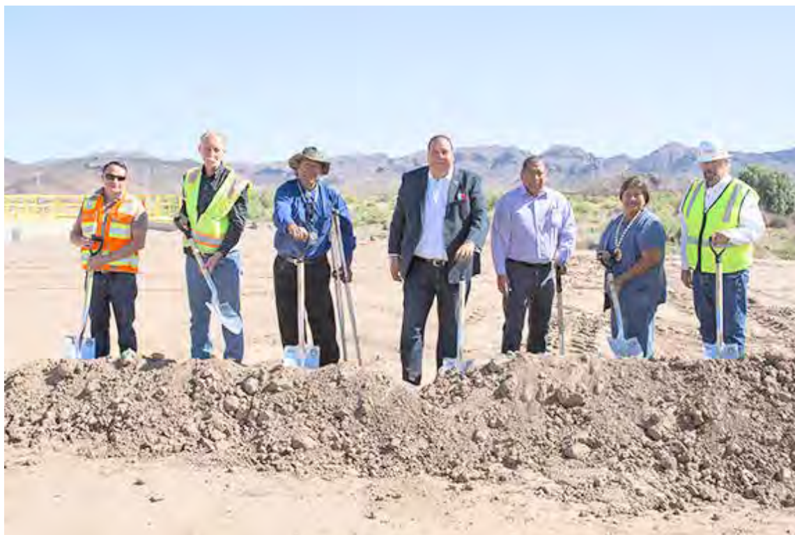
GRIC breaks ground on a new educational preserve at the MAR 5 site on May 14. Christopher Lomahquahu/GRIN
