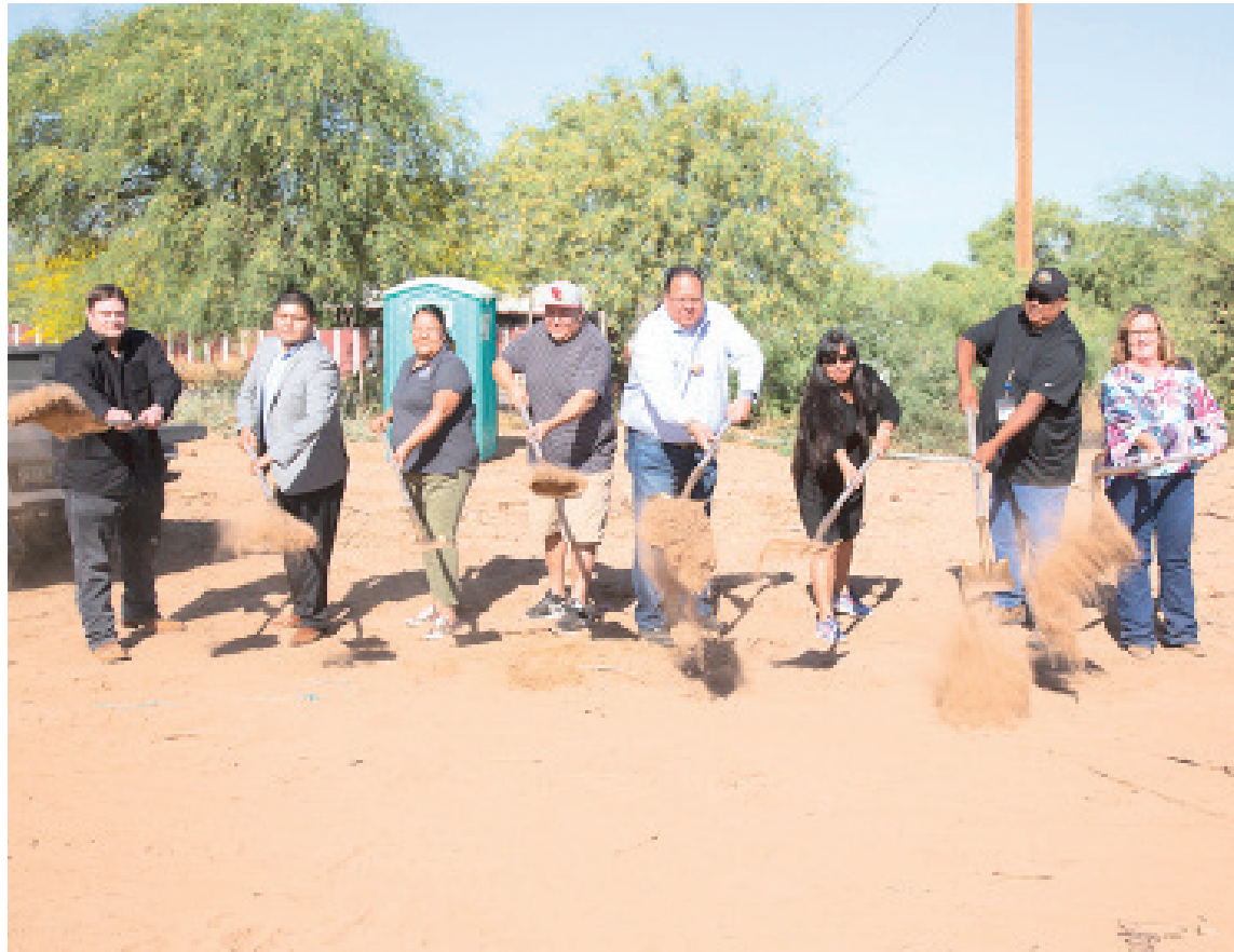
The Gila River Indian Community breaks ground for the 2014 RHIP Housing Project. Aaron J. Tohtsoni/GRIN
