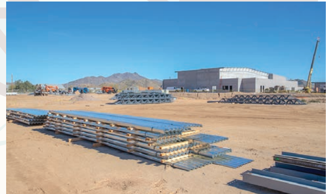
View of the school construction site facing northeast. Roberto A. Jackson/GRIN
