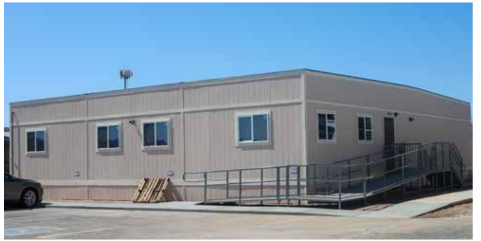
Outside view of the new Genesis building located in District 3 Sacaton across from the GRIC Governance Center. Kyle Knox/GRIN
