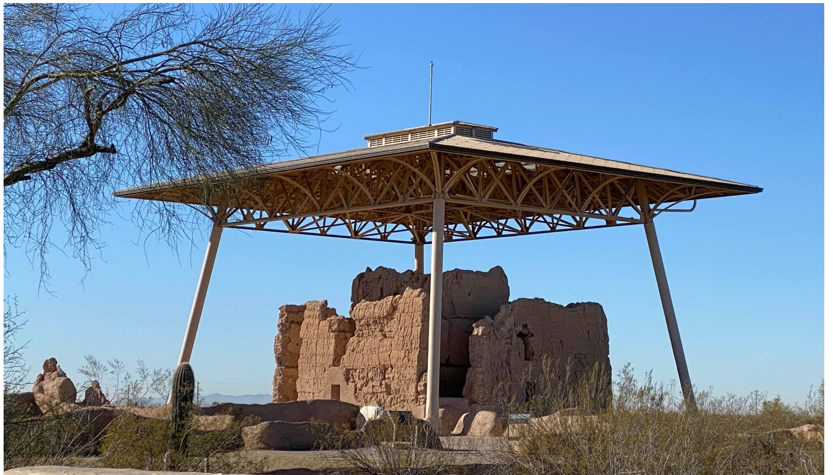
Traditional Trades Apprenticeship Program members will have a chance to work at the site of the large Sivan Vah-Ki “Great House.” Christopher Lomahquahu/GRIN
