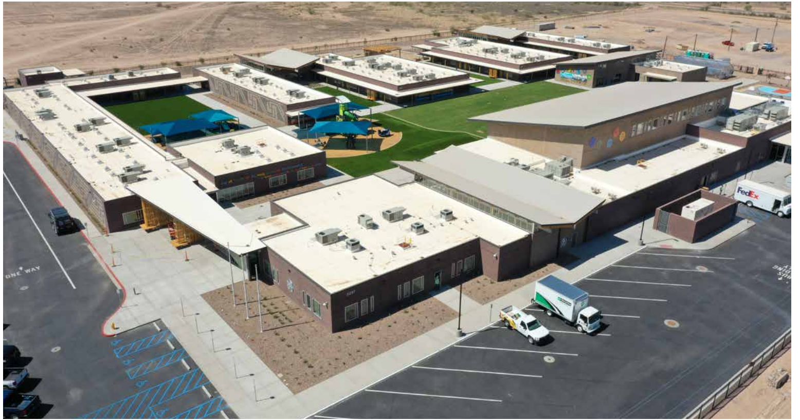
An aerial view of the new Casa Blanca Community School located in District 5. Photo courtesy of Reuben Ringlero
