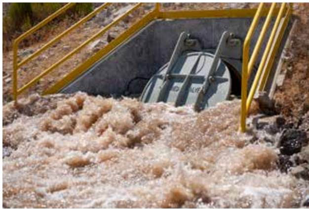
Water used by the Community flows from a release valve at the Managed Aquifer Recharge Site 1B in District 1. Christopher Lomahquahu/GRIN
