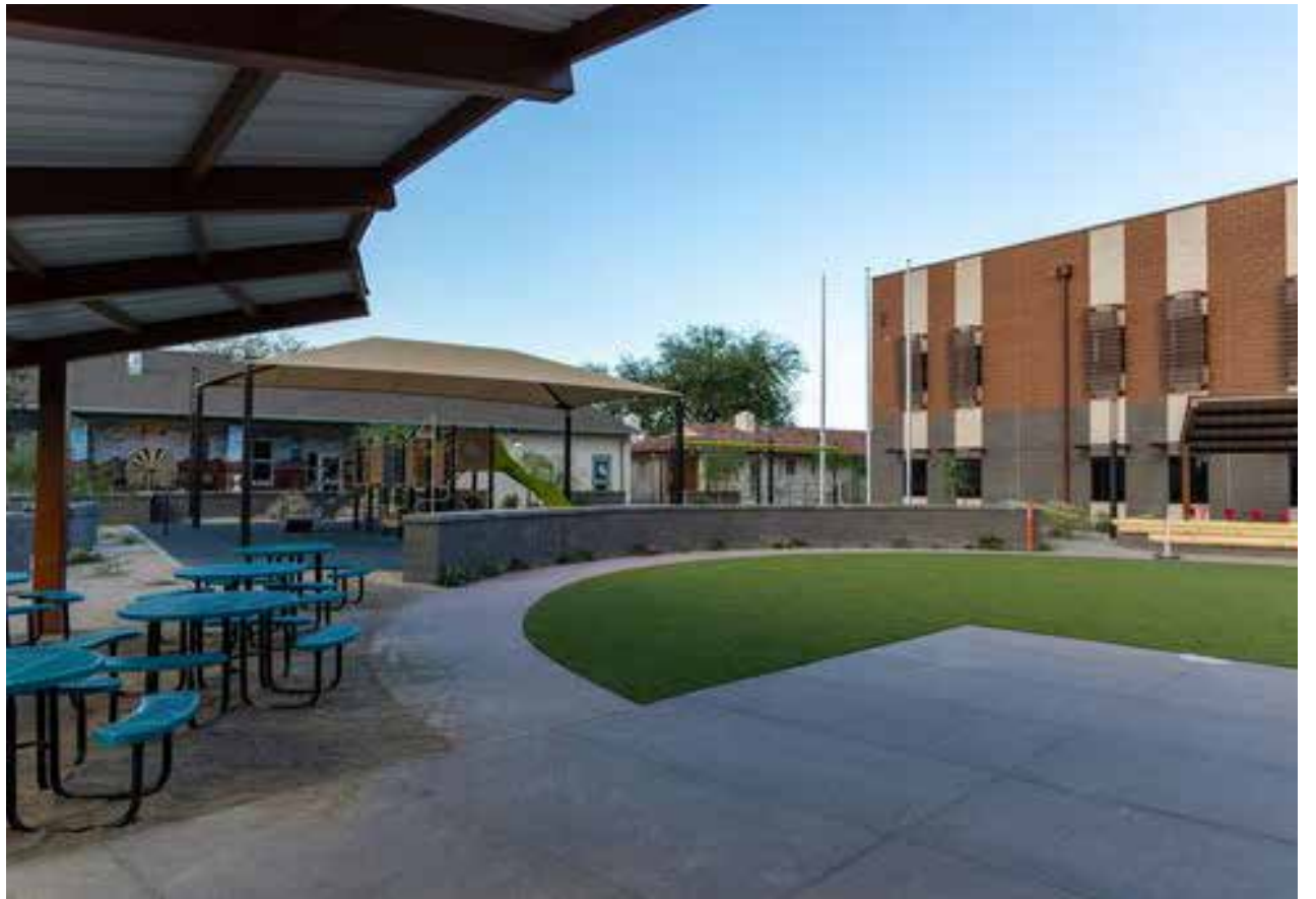
An exterior view of the newly constructed Blackwater Community School, which will replace old school building located next door to the new structure. Photo courtesy of Photos courtesy of Rosendin Electric Company
