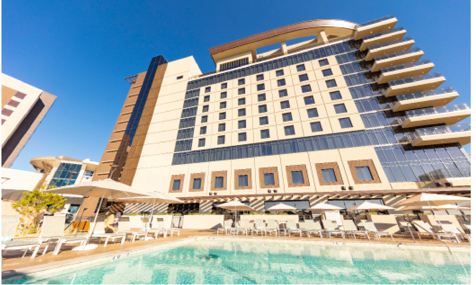
Poolside view of new 11-story Sunrise tower rises 150 feet over the desert landscape. The Sunrise tower features 205 new guest rooms and suites for a total of 447 rooms at Gila River Resorts & Casinos — Wild Horse Pass. Photo courtesy of Point in Time Studios
