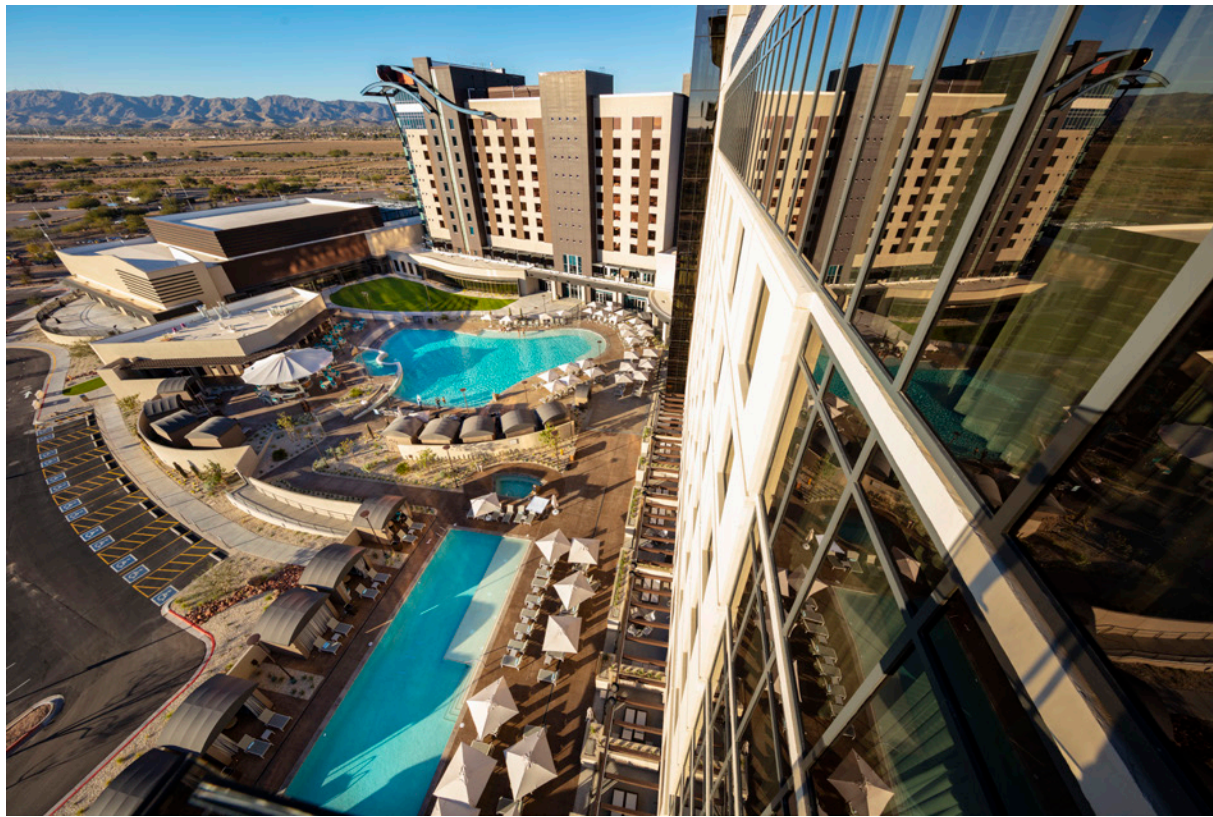
Rooftop view of the new Oasis Pool area that featuring a variety of guest DJ's and performers this summer. Photo courtesy of Gila River Resorts and Casinos
