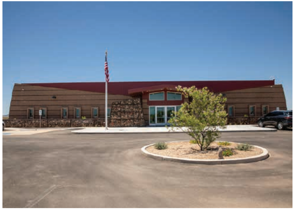
The new sand and gravel building from the front entrance that feature shaded windows to allow in natural lighting while also covering the tops of the windows to prevent sun exposure. Velia Moncada/GRIN
