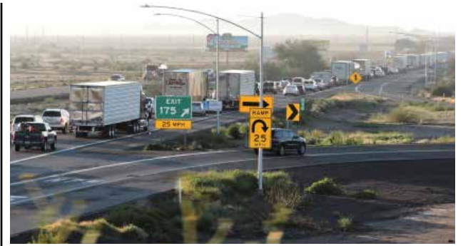
Interstate 10 exit at Casa Blanca Road. Photo Courtesy of Arizona Department of Transportation
