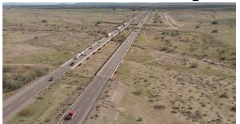
Photo Courtesy of ADOT
