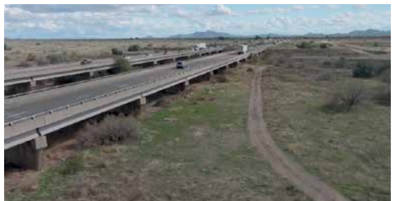
Photo Courtesy of ADOT
